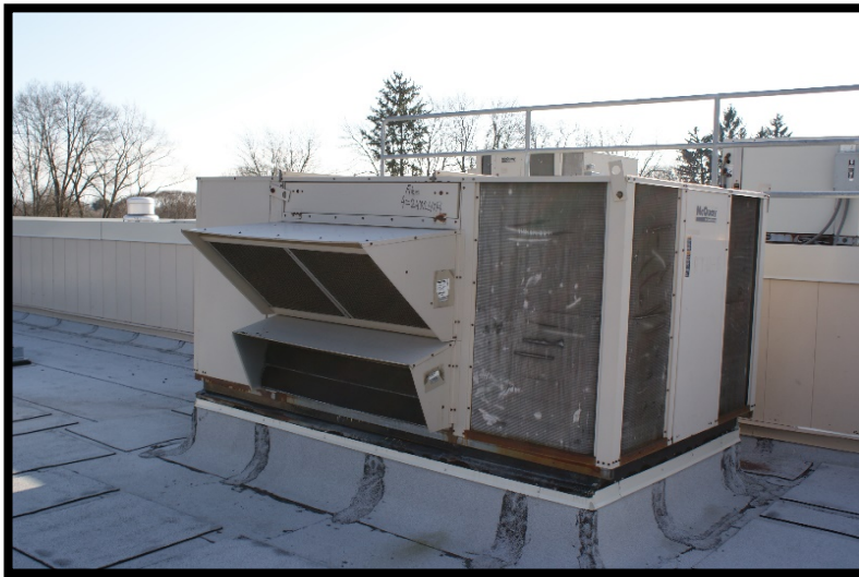
FWMS Replace Main Office HVAC RTU
