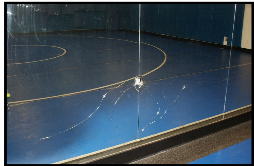
FLHS Yoga Classroom Wall Mirrors Replacement Project
